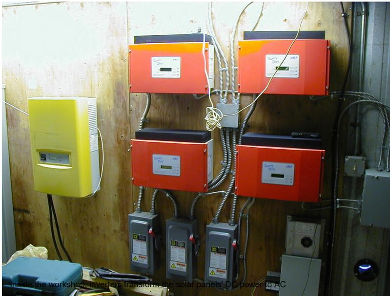
Inside the workshop, inverters transform the solar panels' DC power to AC
